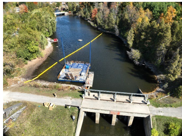
Image 1 - Lanark Dam & barge
