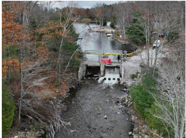
Figure 6. Mazinaw Lake Dam
