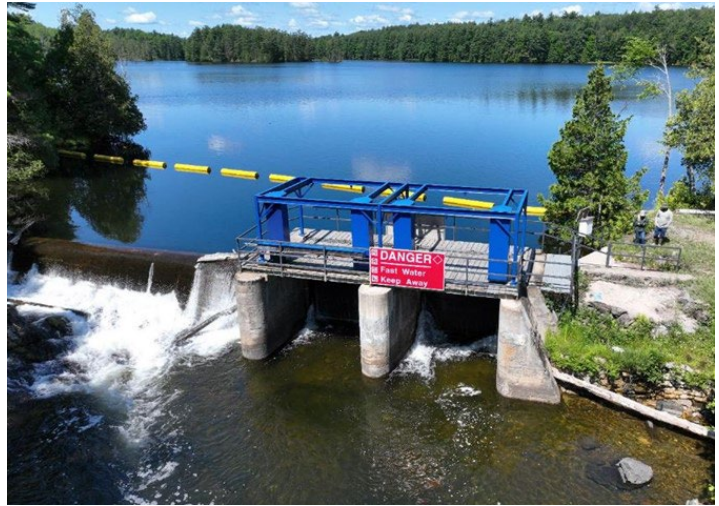
Figure 7. Kashwakamak Lake Dam
