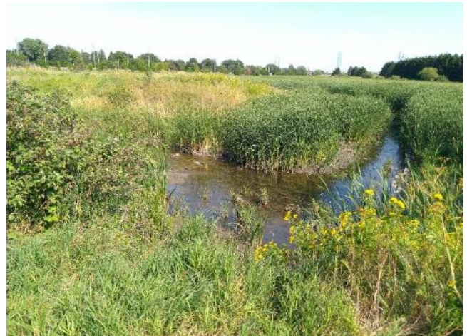
Figure 16. Glen Cairn Flood Control Facility
