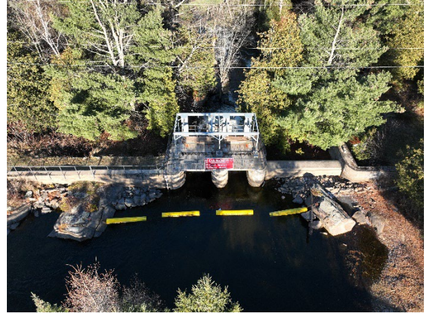
Figure 10. Big Gull Lake Dam
