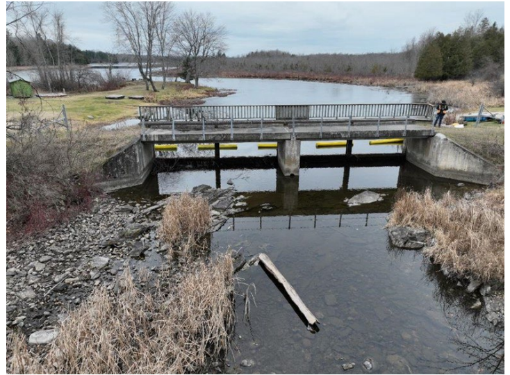
Figure 12. Bennett Lake Dam
