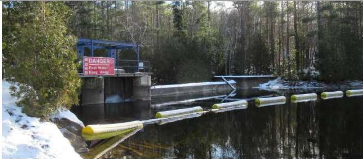
Upstream view of control structure and overflow weir.
