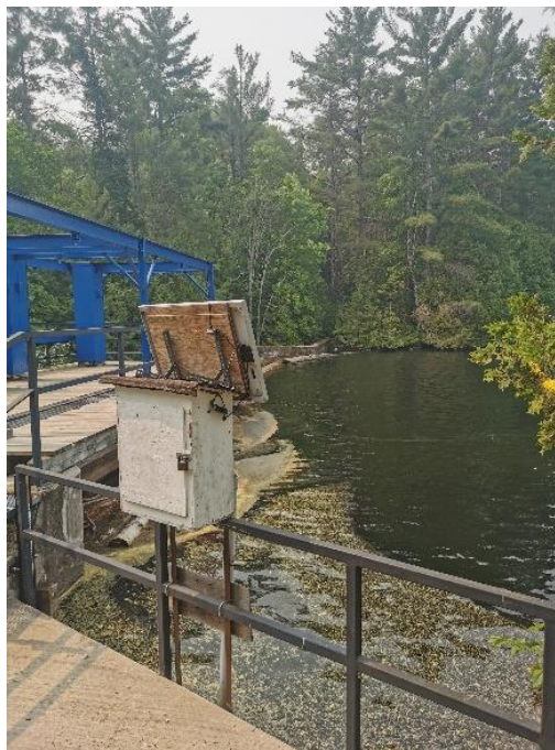
Figure 10: Kashwakamak Lake Dam, sluiceway and deck, looking north.
