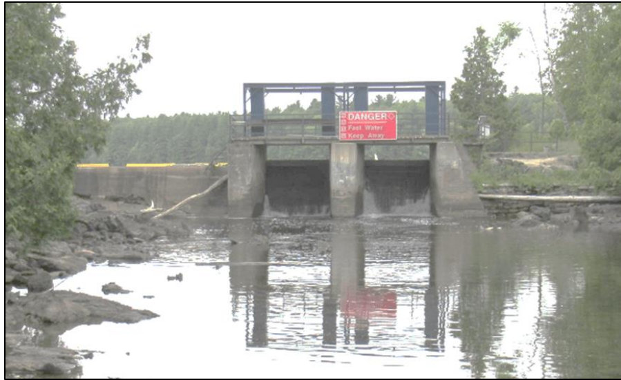
Image 1. Photograph of the Kashwakamak Lake Dam, facing west-northwest. (Courtesy of MVCA)
