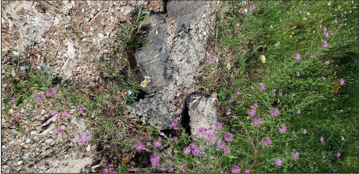
Image 9. View of a secondary patch of concrete fill at the northern end of the control dam, facing east. (PR23-021D014)
