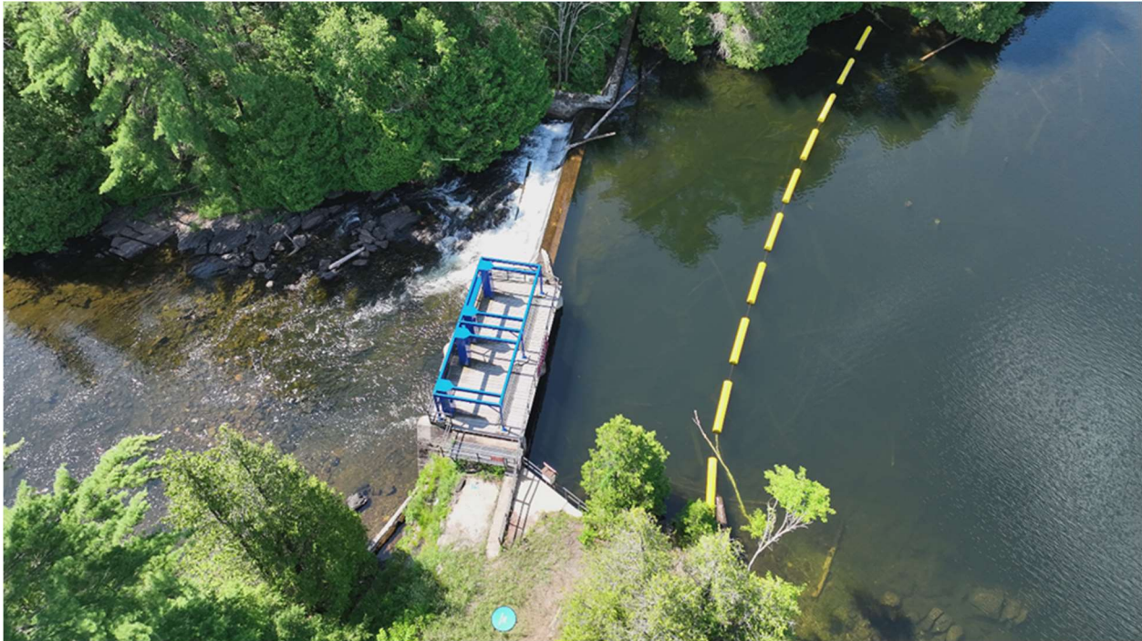
Figure 4: MVCA Drone Photo (07/19/2023)
