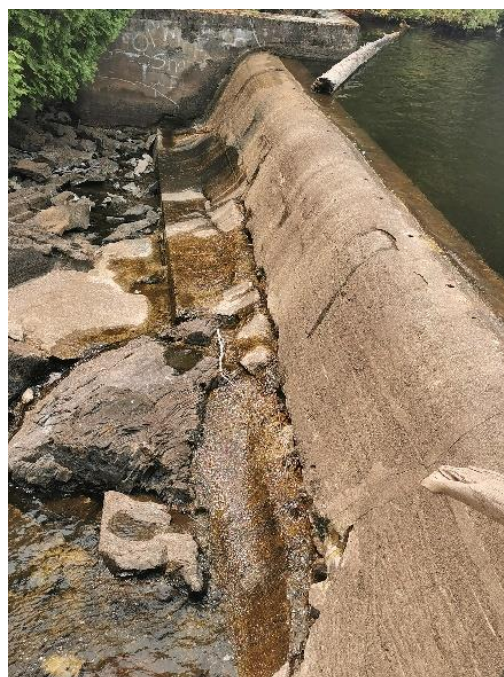
Figure 12: Kashwakamak Lake Dam, spillway detail.
