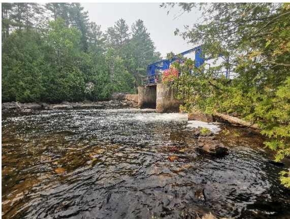
Figure 5: Kashwakamak Lake Dam, looking northwest.
