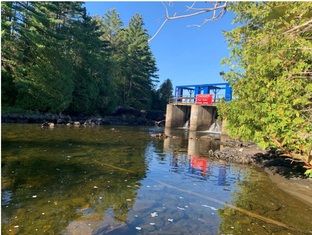
Image 5: Sluiceway from downstream site facing southwest.
