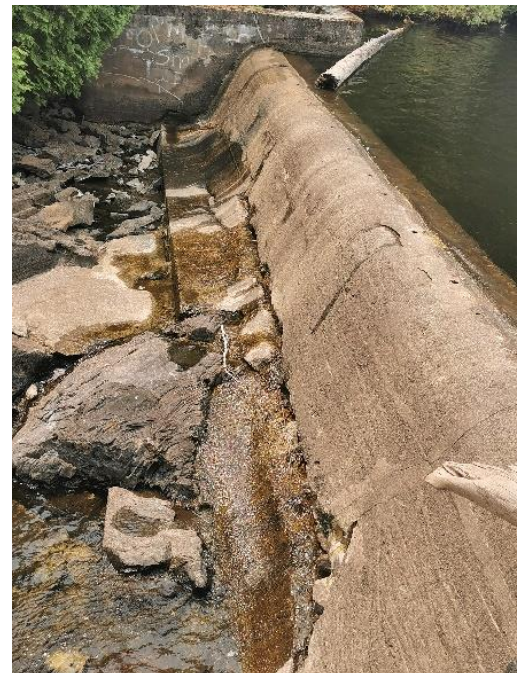
Figure 12: Kashwakamak Lake Dam, spillway detail.
