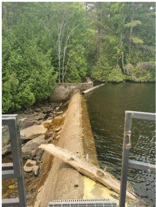
Figure 9: Kashwakamak Lake Dam, overflow spillway.
