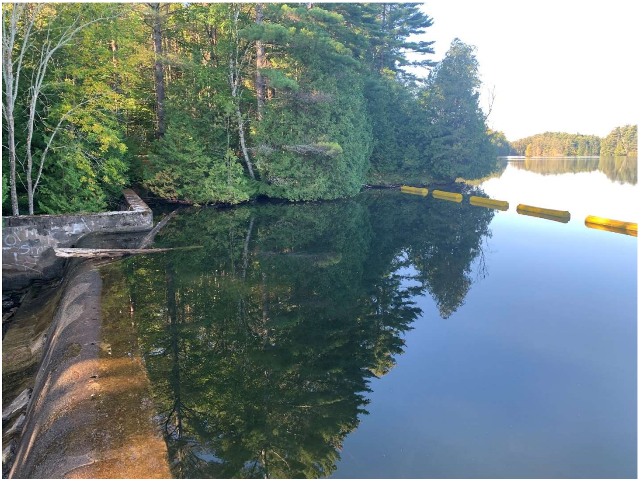
Image 4: Overflow dam and south wingwall facing southwest.
