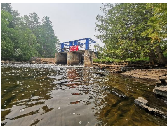
Figure 7: Kashwakamak Lake Dam, looking west.
