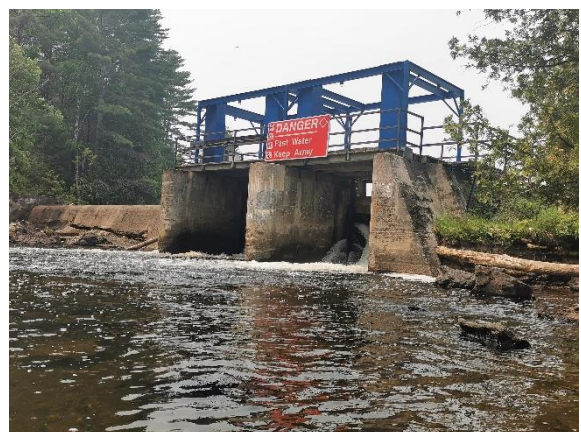
Figure 8: Kashwakamak Lake Dam, sluiceway and overflow looking west.
