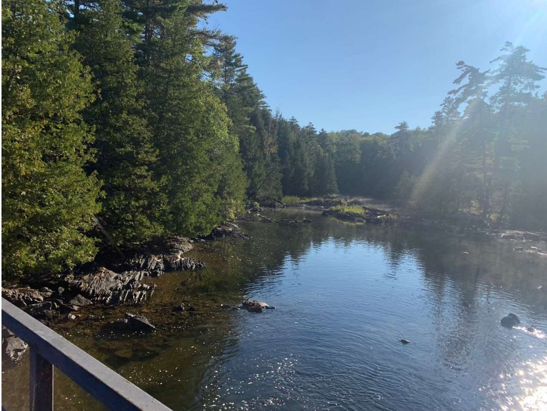
Image 6: Downstream from top of dam structure facing east.
