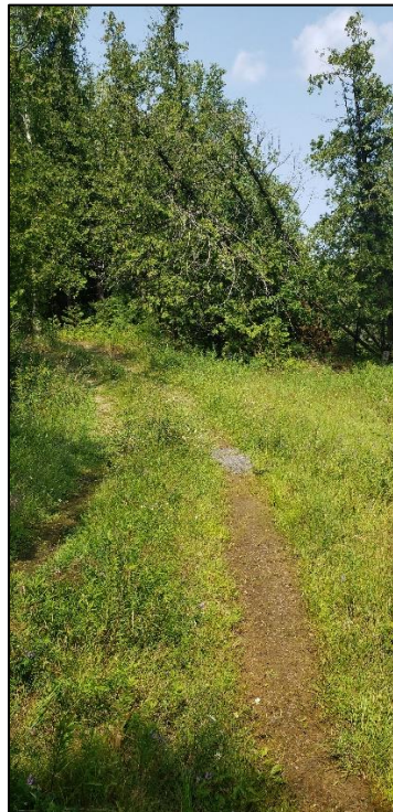
Image 16. View of the access road near the saddle dam, facing north. (PR23-021D044)
