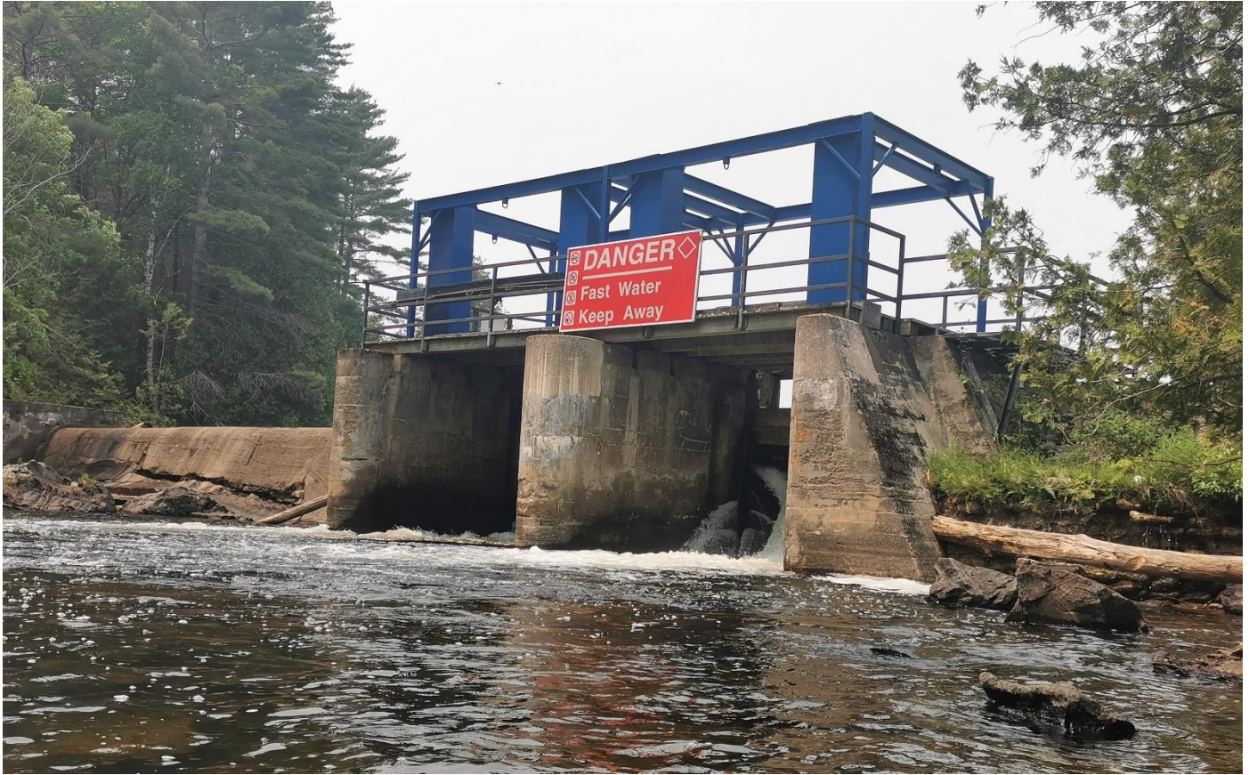
Kashwakamak Lake Dam, Mississippi River, Township of North Frontenac
