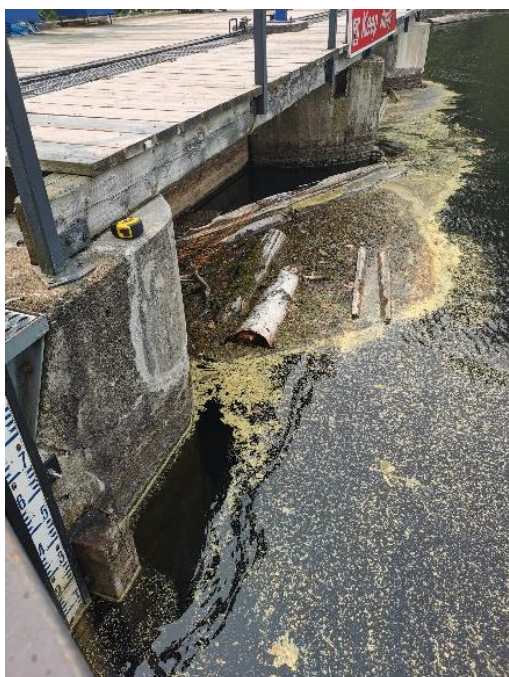
Figure 11: Kashwakamak Lake Dam, sluiceway and deck, detail.
