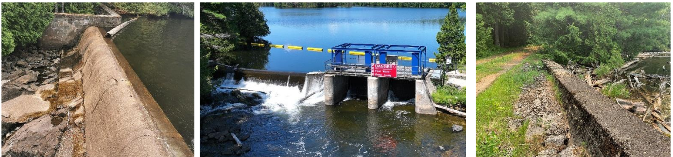
Photos: Overflow weir of main dam (left), Kashwakamak Lake Dam (overflow weir and two sluices gates, middle), and saddle dam (right).
