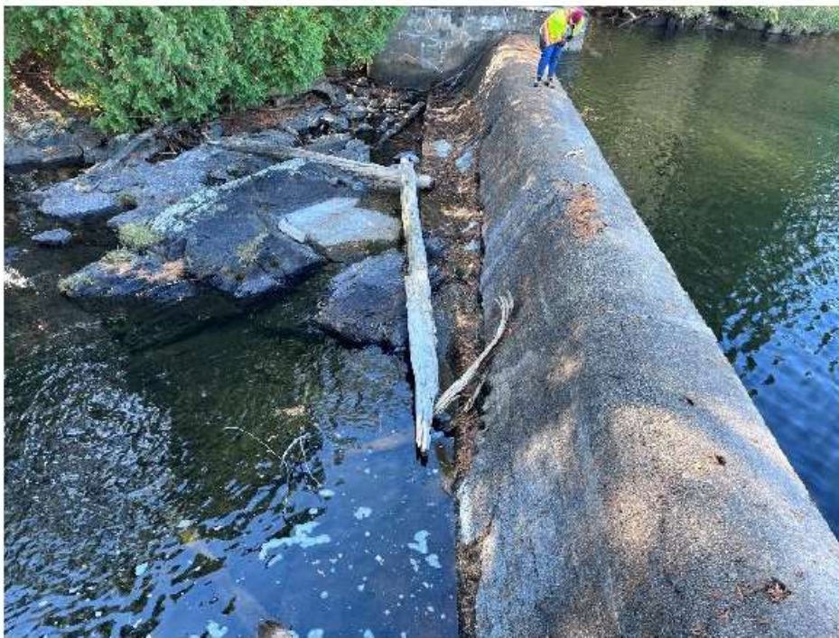
View of the overflow weir.
