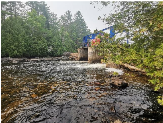
Figure 5: Kashwakamak Lake Dam, looking northwest.
