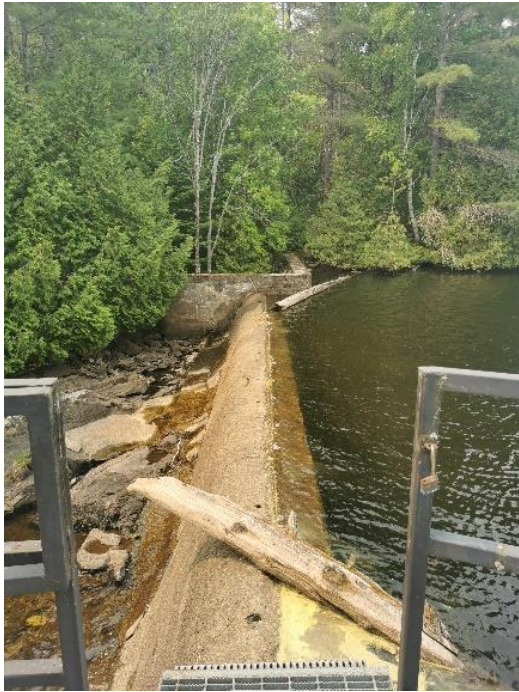
Figure 9: Kashwakamak Lake Dam, overflow spillway.
