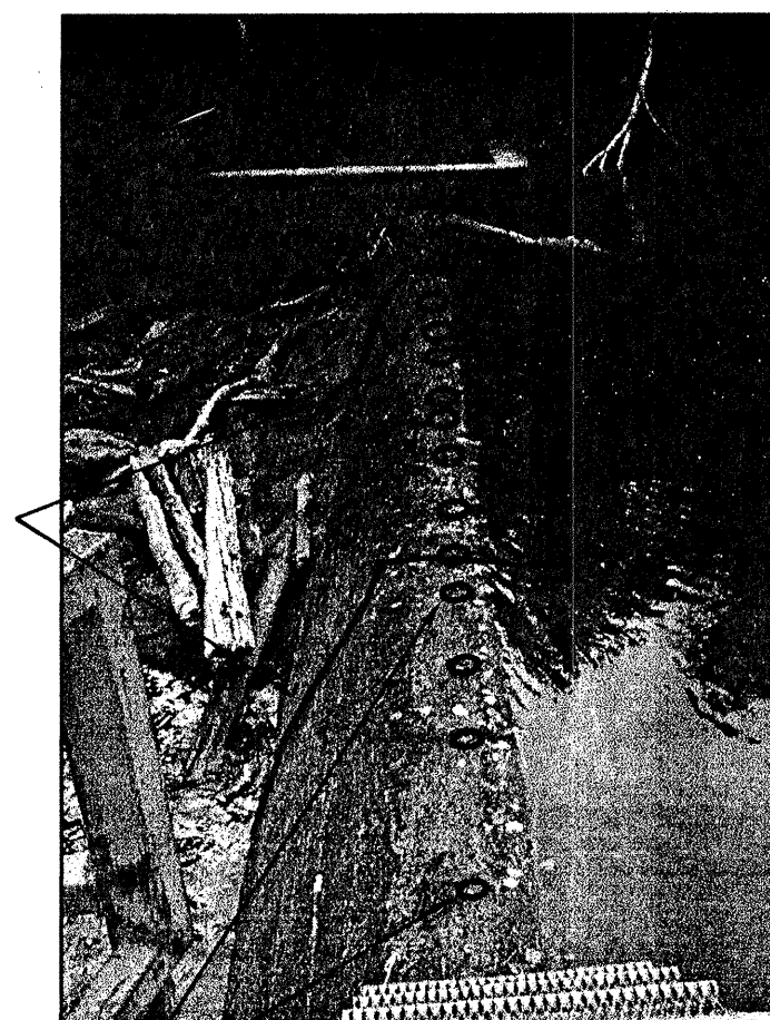
ABANDONED POST HOLES FOR FLASHBOARDS
