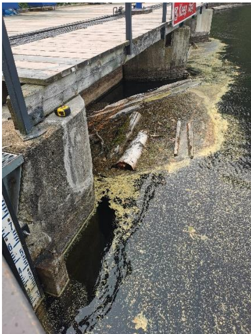
Figure 11: Kashwakamak Lake Dam, sluiceway and deck, detail.
