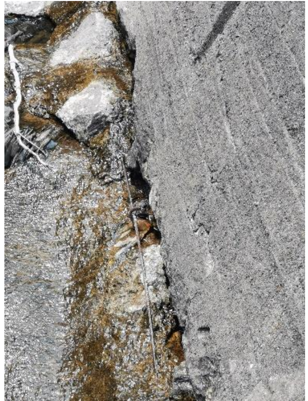
Figure 14: Kashwakamak Lake Dam, concrete detail.
