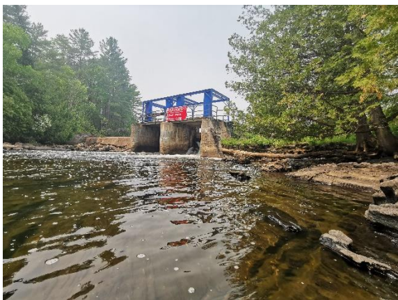
Figure 7: Kashwakamak Lake Dam, looking west.
