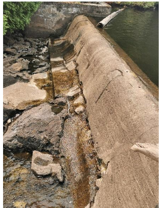
Figure 12: Kashwakamak Lake Dam, spillway detail.
