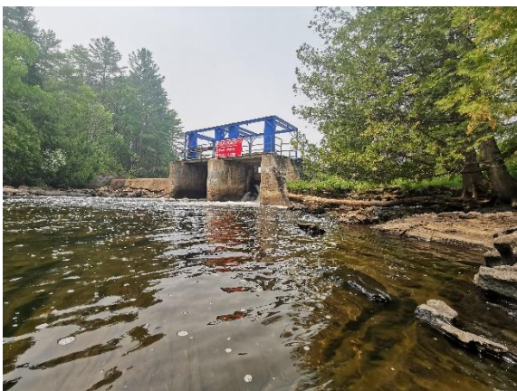
Figure 7: Kashwakamak Lake Dam, looking west.
