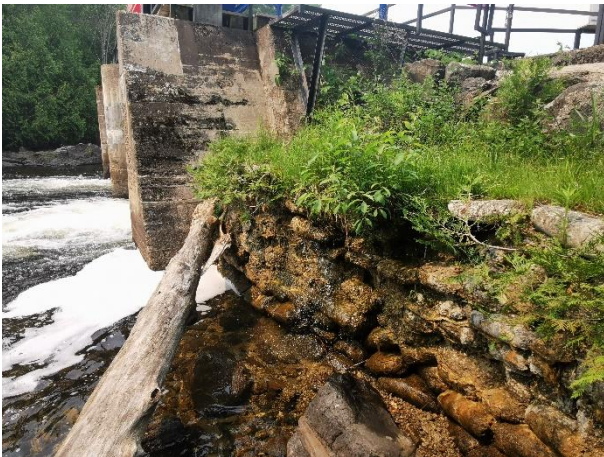
Figure 13: Kashwakamak Lake Dam, left concrete abutment and earthen embankment.
