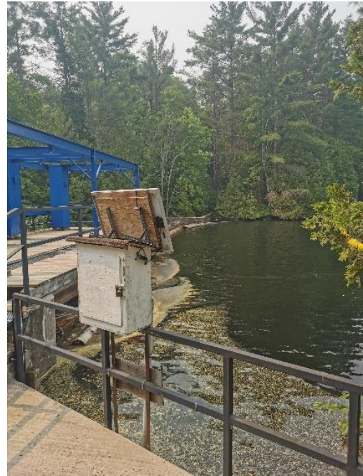
Figure 10: Kashwakamak Lake Dam, sluiceway and deck, looking north.
