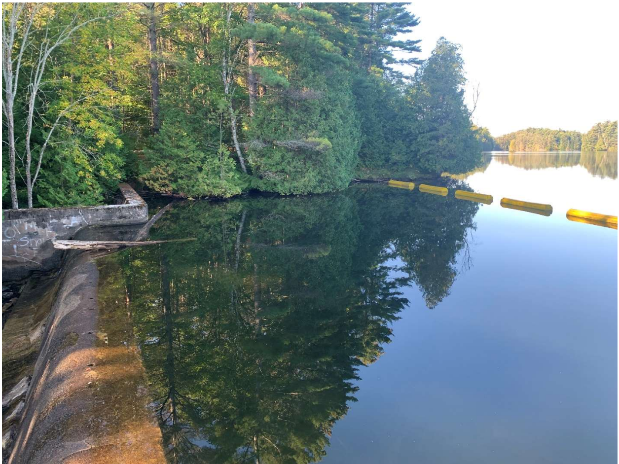
Image 4: Overflow dam and south wingwall facing southwest.
