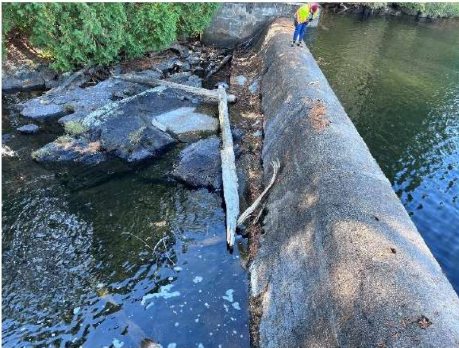
View of the overflow weir.
