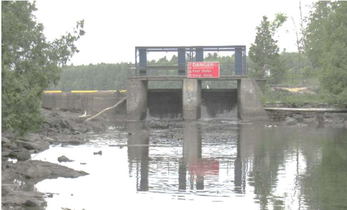
Image 1: Main control dam (MVCA 2023)
