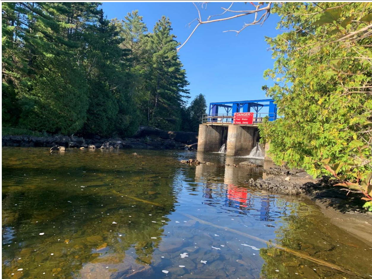
Image 5: Sluiceway from downstream site facing southwest.
