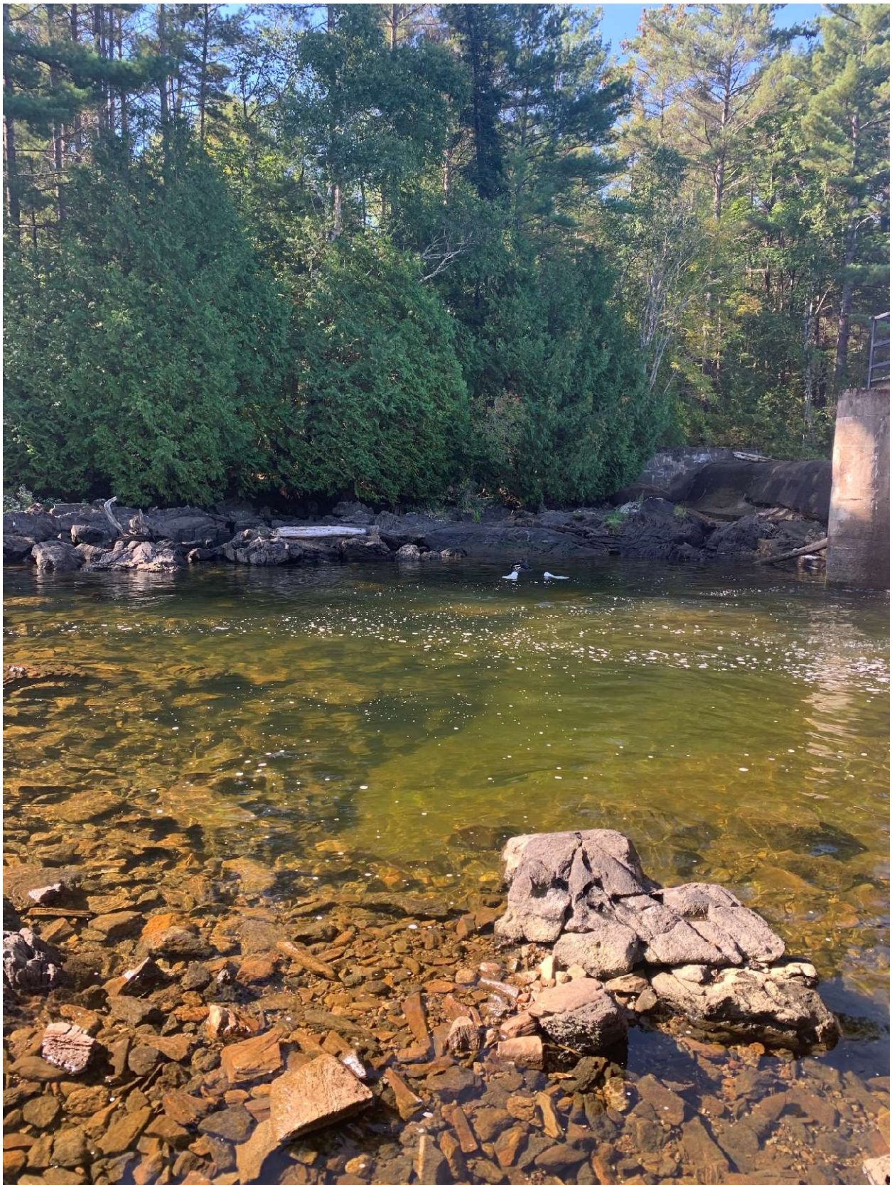
Image 12: Snorkel Survey near south wingwall and plunge pool
