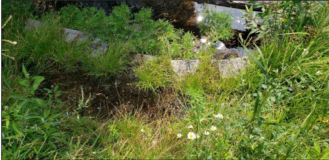
Image 7. View from above of the retaining wall at the north end of the control dam, facing east. (PR23-021D013)
