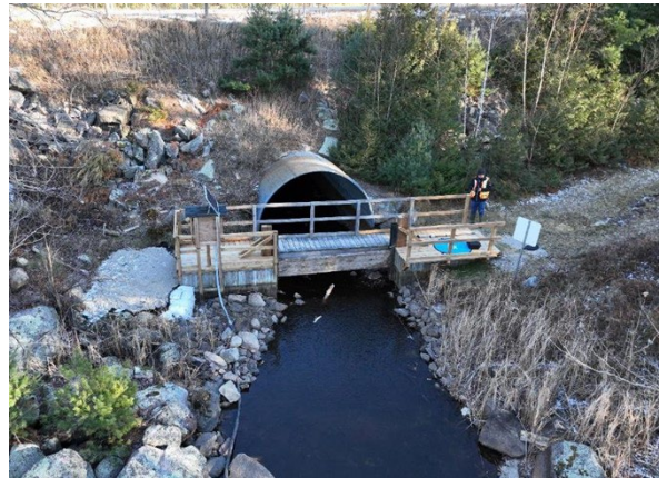
Figure 11. Pine Lake Dam
