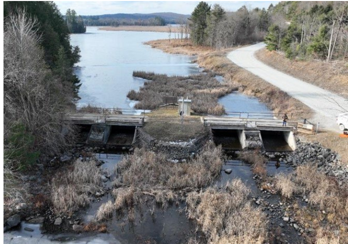
Figure 13. Widow Lake Dam
