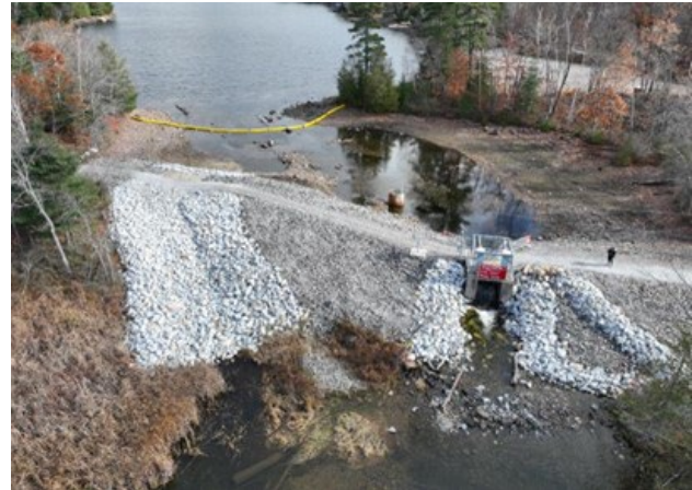
Figure 5. Shabomeka Lake Dam
