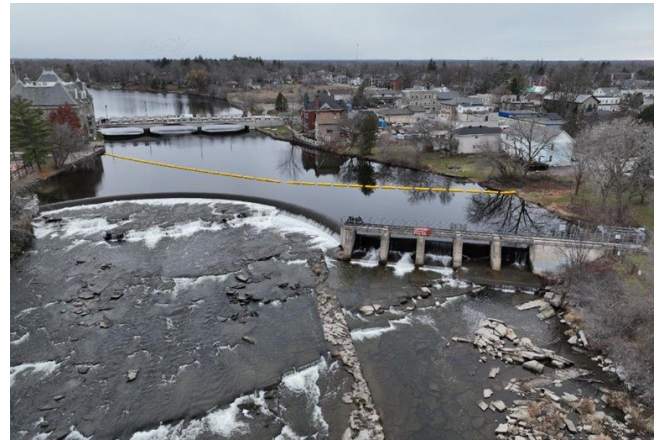
Figure 15. Carleton Place Dam
