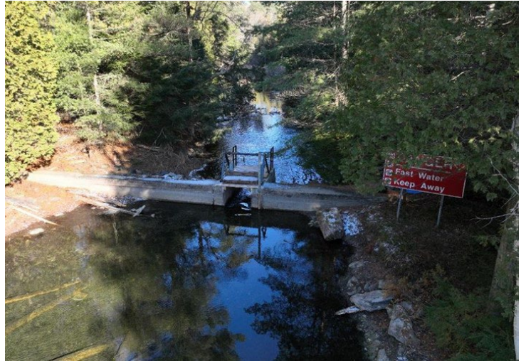
Figure 8. Mississagagon Lake Dam
