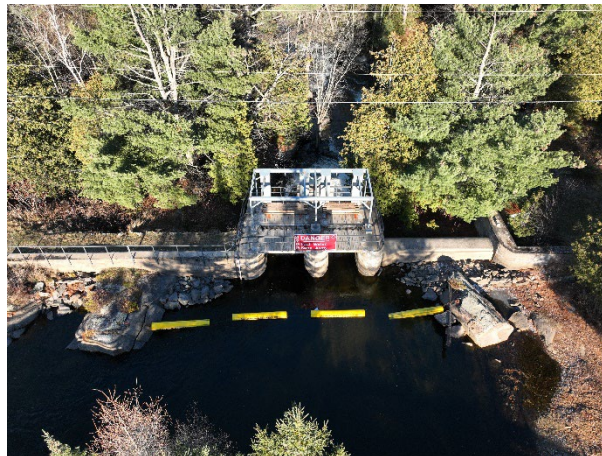
Figure 10. Big Gull Lake Dam
