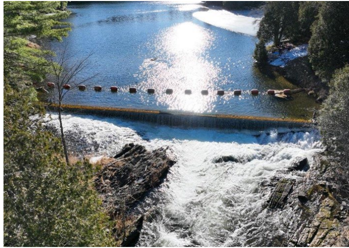
Figure 9. Farm Lake Dam
