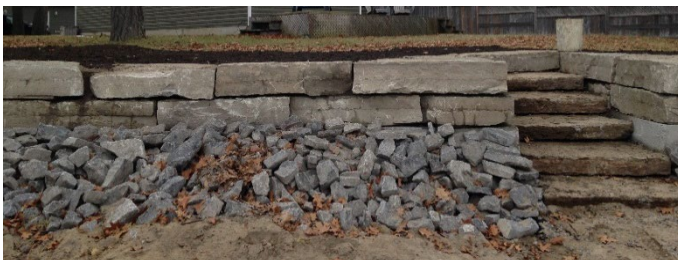
Armour Stone Wall with Rip Rap
