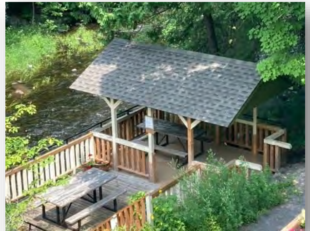
Mill of Kintail lookout, new roof
