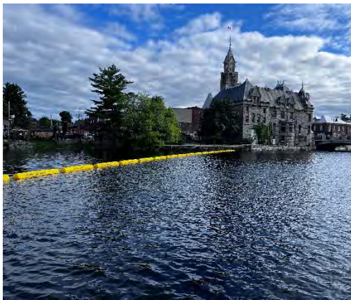
Carleton Place Dam Boom Replacement
