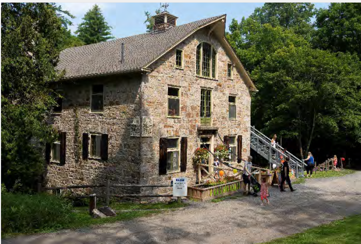
Mill of Kintail Museum, new roof
