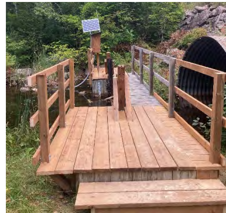
Pine Lake Dam Safety Controls
