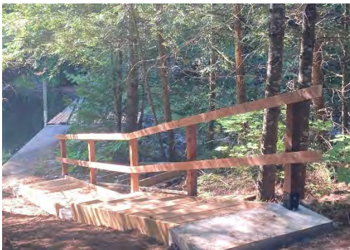
Mississagagon Lake Dam, railing installation
