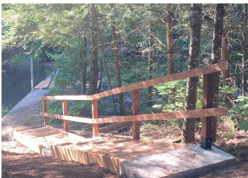
Mississagagon Lake Dam, railing installation
