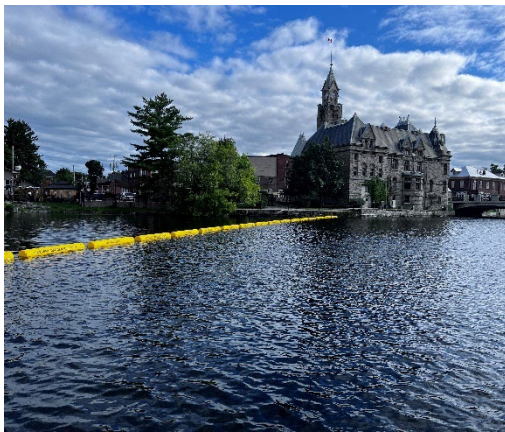
Carleton Place Dam Boom Replacement
