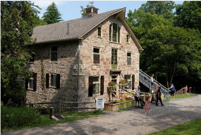
Mill of Kintail Museum, new roof
