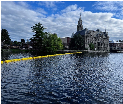
Carleton Place Dam Boom Replacement
