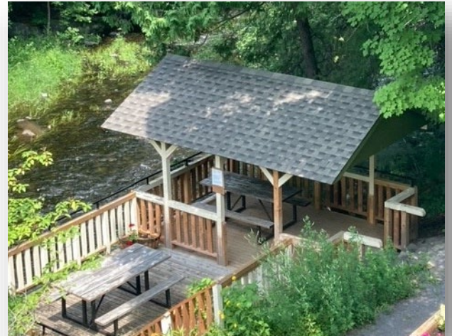
Mill of Kintail lookout, new roof
