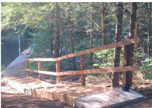
Mississagagon Lake Dam, railing installation
