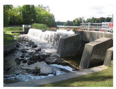
The purpose of the dam is to maintain recreational water levels on Clayton and Taylor Lakes, combined with low flow augmentation of the downstream river system. MVCA has historic experience<sup>3</sup> with this dam and has no concerns with assuming responsibility for its operation.
