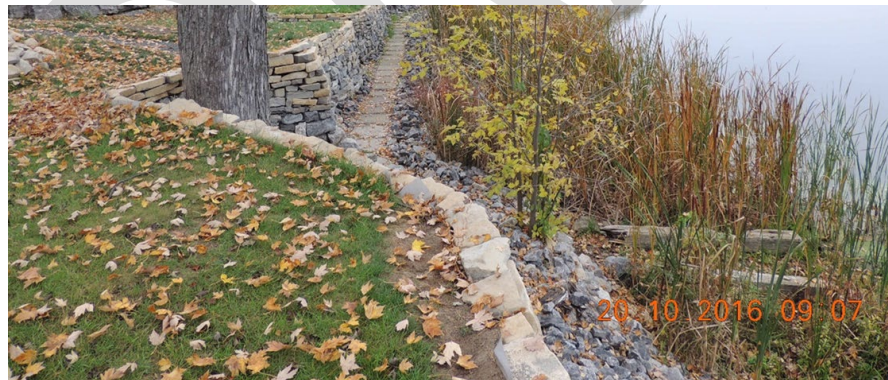
Erosion protection incorporating vegetation along shoreline.
