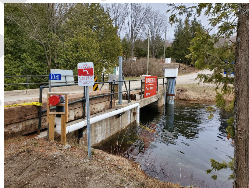
Dry hydrant at Palmerston Lake Dam
