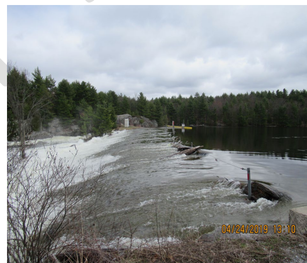
Overtopping of Crotch Lake Weir, Spring 2019
