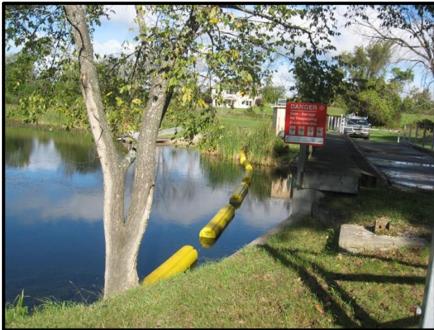
Bennett Lake Dam
