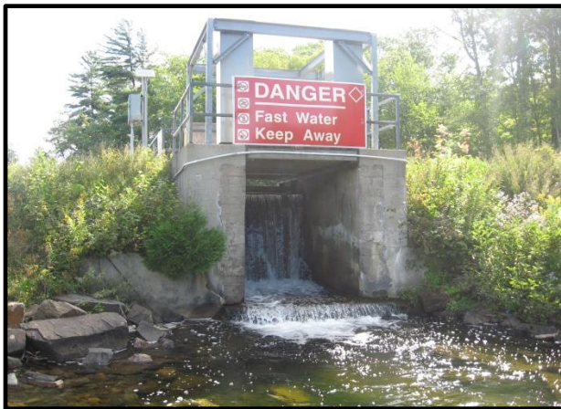
Shabomeka Lake Dam
