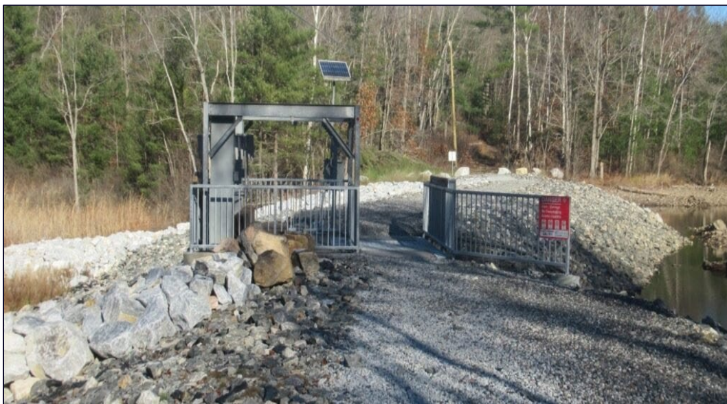
Recently rehabilitated Shabomeka Lake Dam deck and embankment with new safety railing
