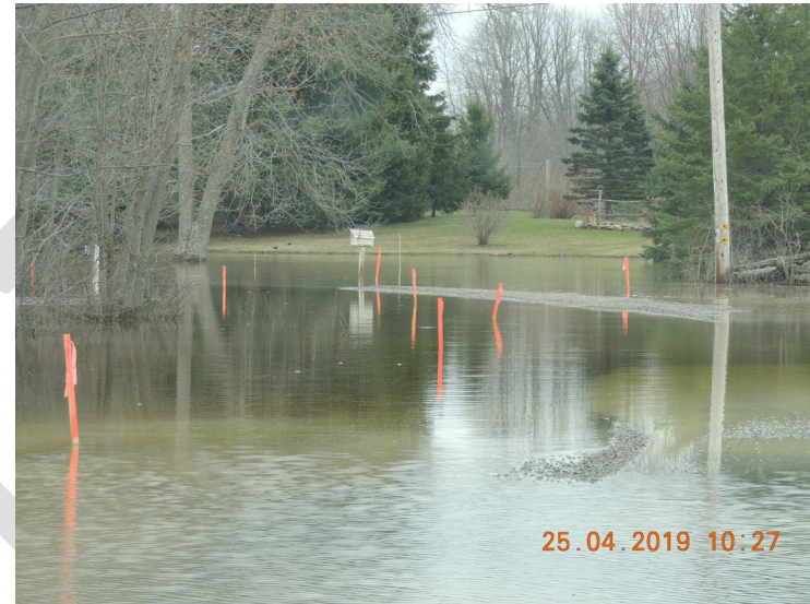
Flooding of a private road - Mississippi Lake, Spring 2019
