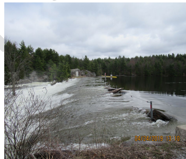
Overtopping of Crotch Lake Weir, Spring 2019
