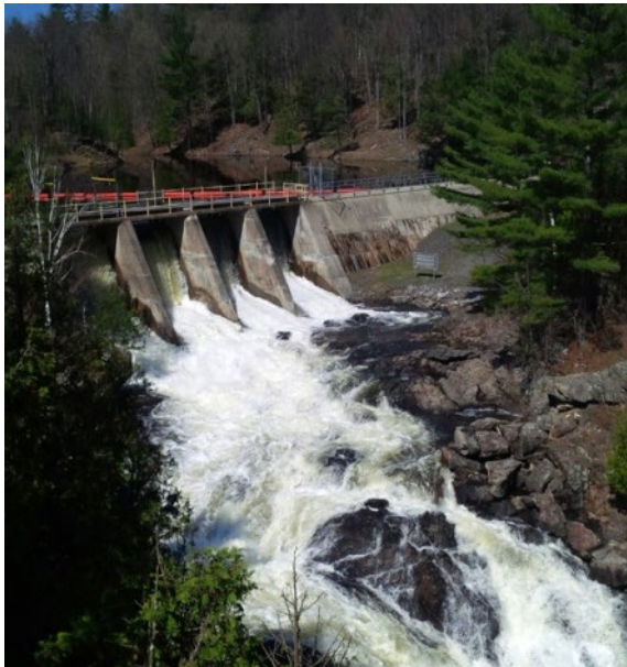
High Falls Diversion Dam
