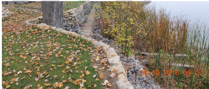
Erosion protection incorporating vegetation along shoreline.
