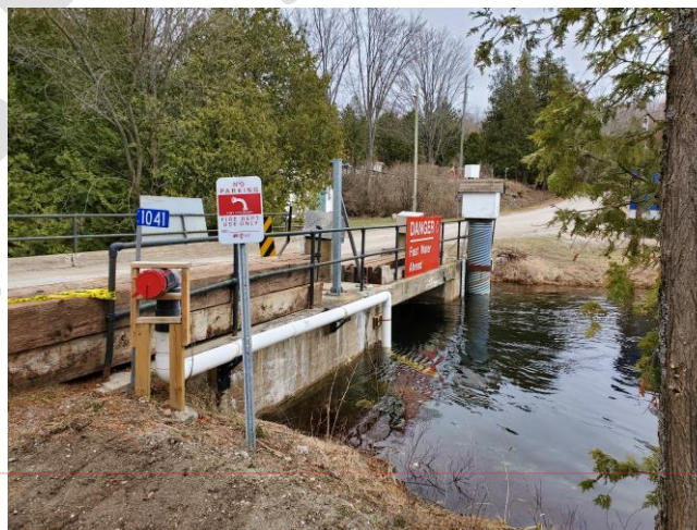
Dry hydrant at Palmerston Lake Dam
