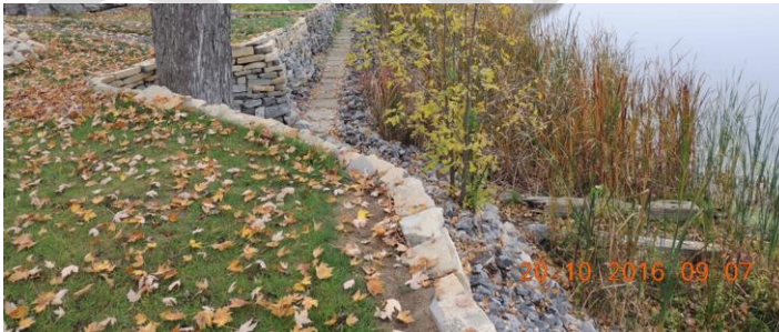
Erosion protection incorporating vegetation along shoreline.
