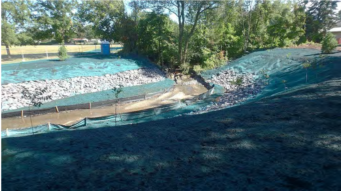
Realignment and shoreline stabilization of the upper Carp River, Kanata.
