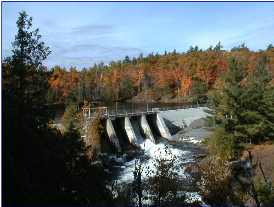
High Falls Generating Station – Mississippi River, Ontario
