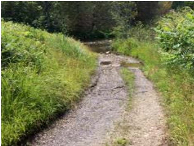
ATV trail to stream crossing south of dam. Note seepage along edge of berm.
