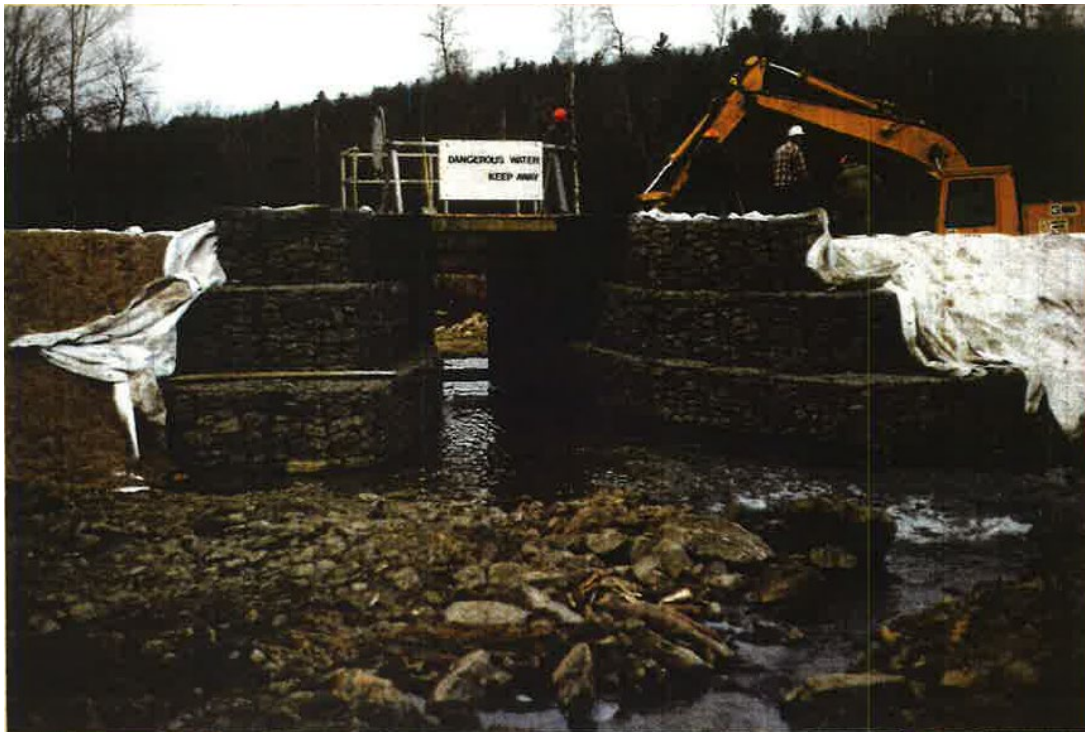
Figure 20: View of new embankment sand and gabion walls, 1989 (MCVA, 2005).
