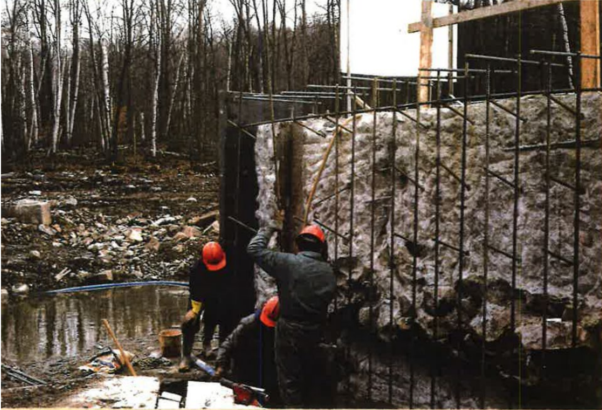
Figure 17: Formwork for new concrete portions of concrete sluice in 1989 (MCVA, 2005).
