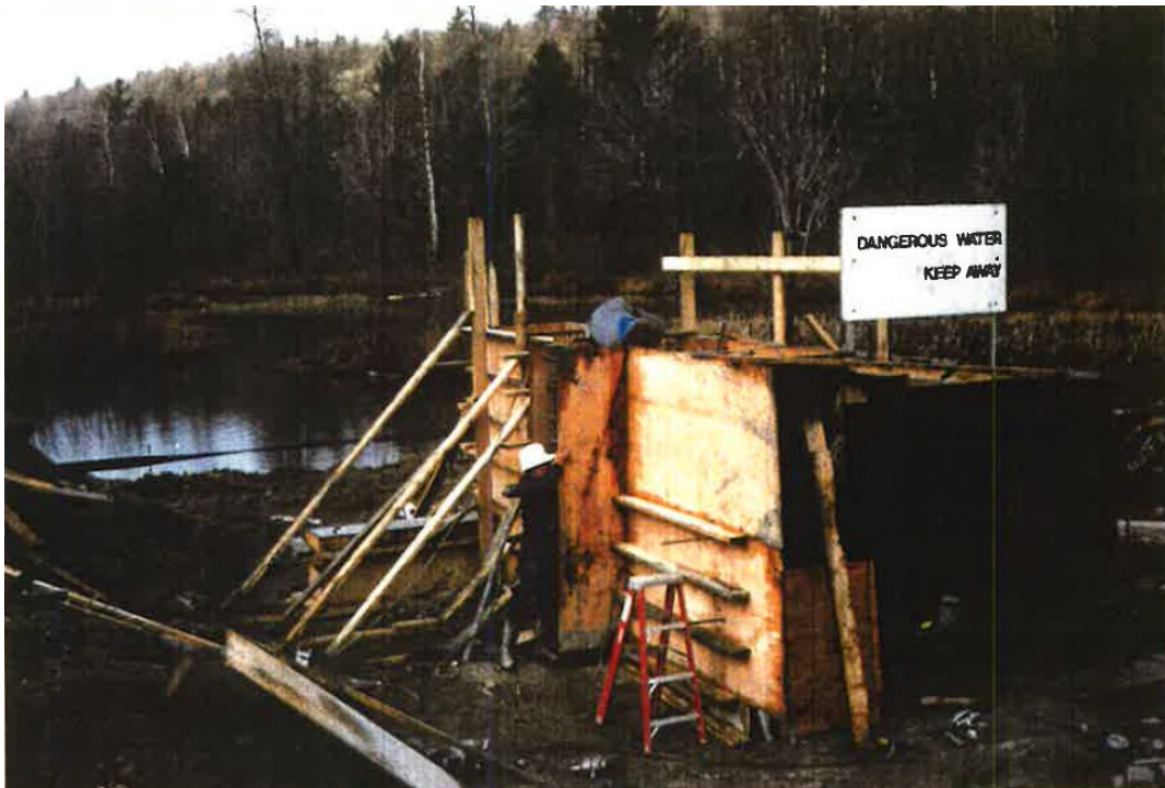
Figure 16: Formwork for new concrete sluice walls in 1989 (MCVA, 2005).
