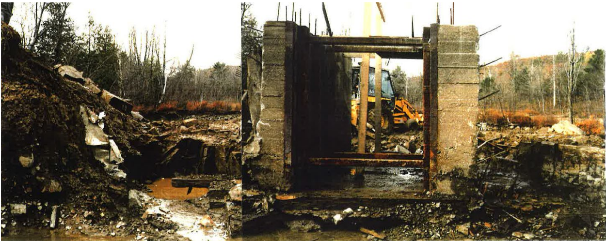
Figure 18: Sluiceway pre-1989 reconstruction, showing partial removal of embankments (MCVA, 2005).
