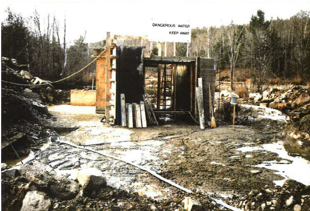
Figure 19: Upstream view of 1989 reconstruction showing embankments removed (MCVA, 2005).
