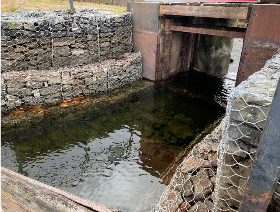
Figure 8: Rock shoring on all sides of the dam (CU 2019).
