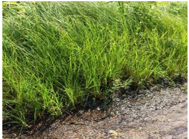
Seepage along front edge of north berm. Note wetland vegetation (sedges).
