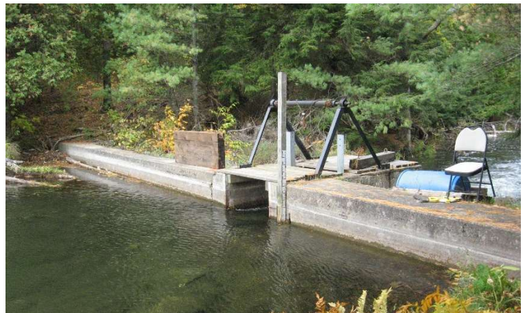
The dam and gauge at the outlet of Mississagagon Lake
