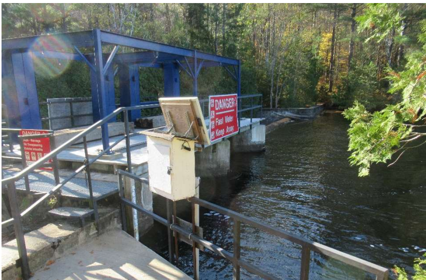
The dam and gauge station at the outlet of Kashwakamak Lake
