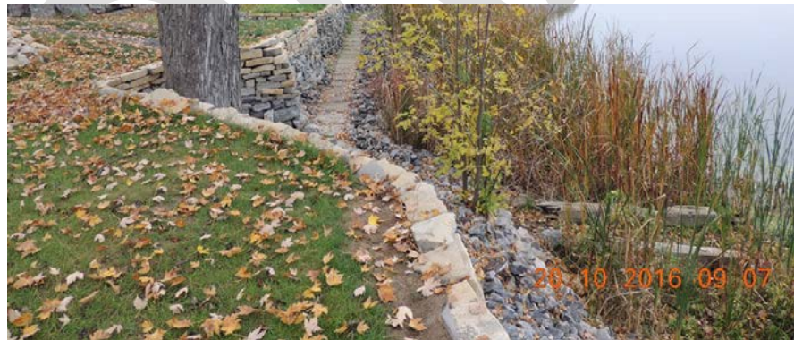
Erosion protection incorporating vegetation along shoreline.
