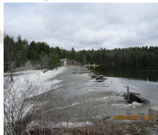
Overtopping of Crotch Lake Weir, Spring 2019
