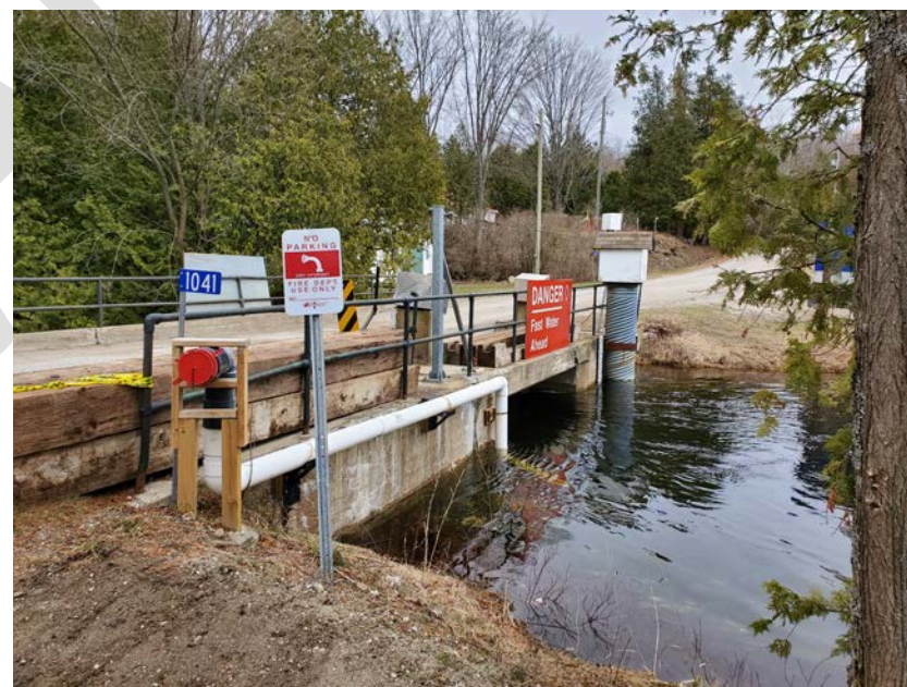
Dry hydrant at Palmerston Lake Dam
