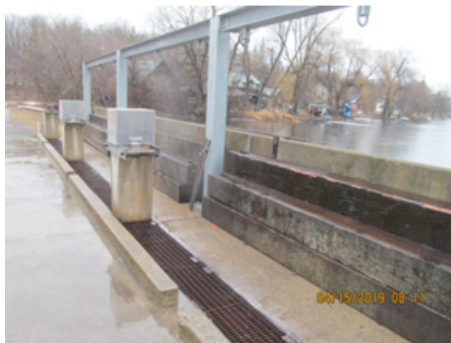
Photo 48 Stoplogs on Lanark Dam
