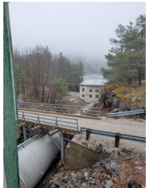
Photo 30 - High Falls G.S. Penstock & Powerhouse
