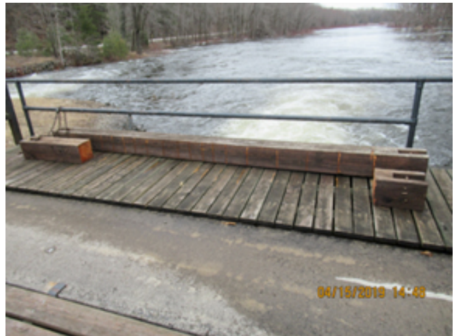
Photo 46 Vandalism of stoplogs at Widow Lake Dam
