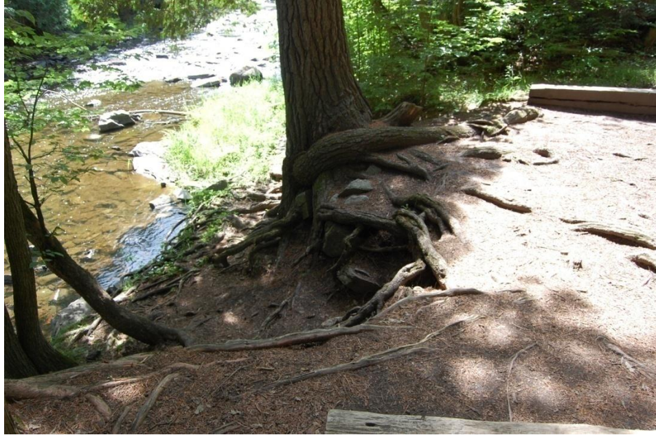
Heavily eroded riverbank
